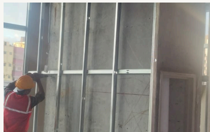
Perimeter partition framing
