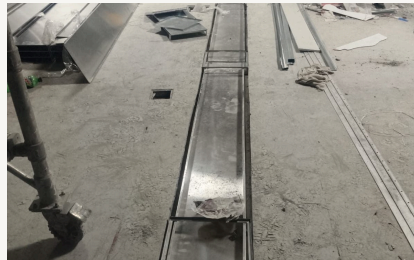
Partition track setting out
