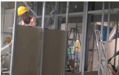
Gypsum board fixing
