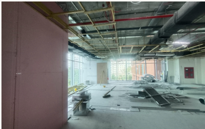
Bare shell before fit-out
